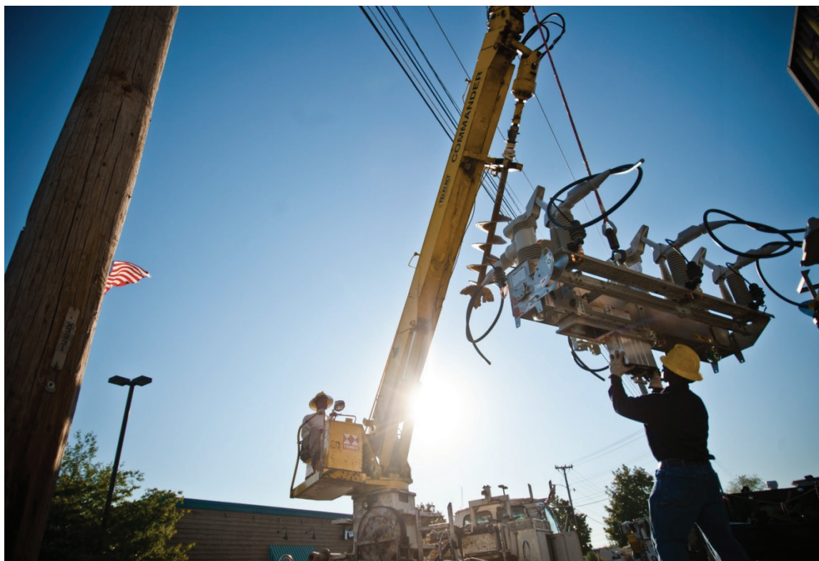
FIGURE 4-18 Installation of an IntelliRupter Pulse Closer. SOURCE: McCarthy, 2015. Image courtesy of POWERGRID International.
